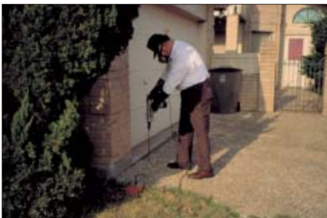
A rotary hammer drill is used to drill holes for the sub-slab method of termite treatment.
