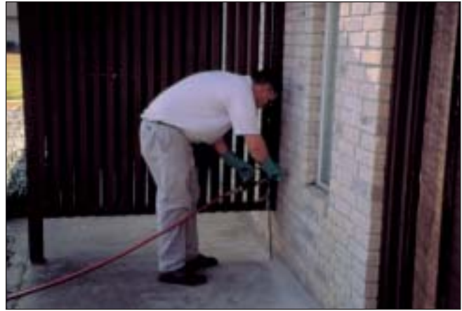
Termiticide is injected in drill holes.
