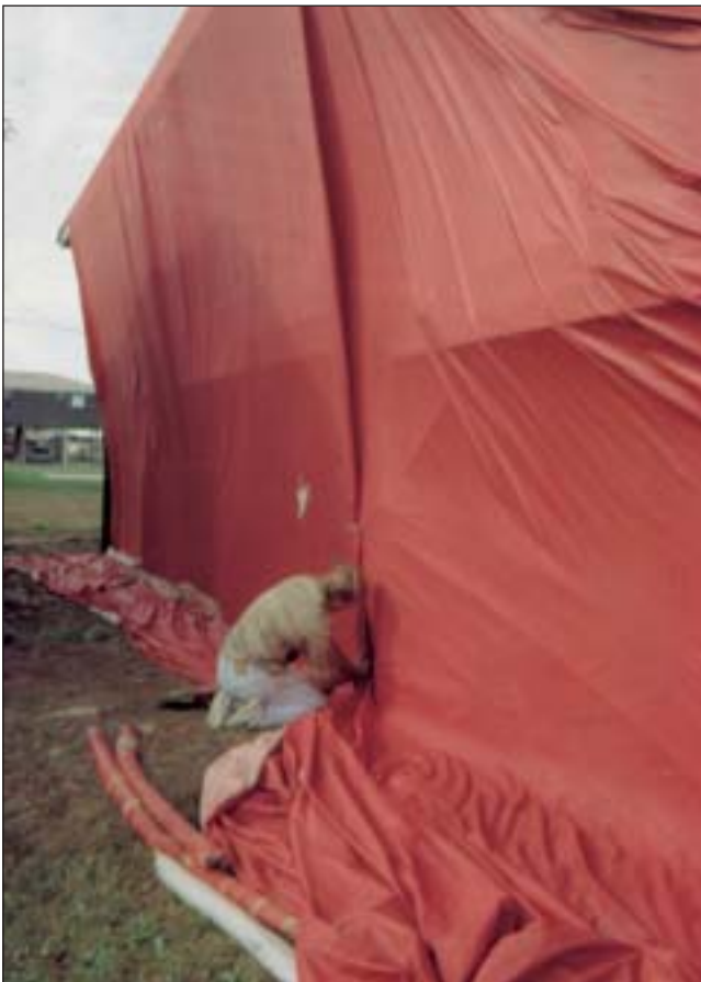
Fumigation is used to treat drywood termites.
